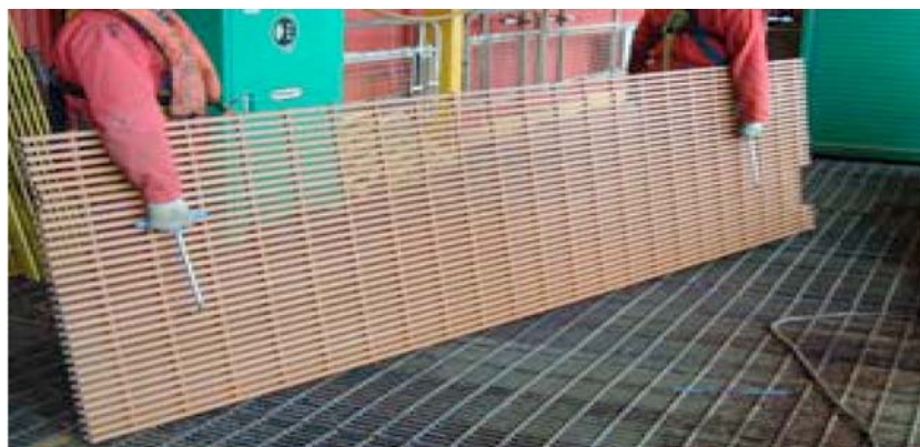
FIG. X1.14 Correct Handling of FRP Gratings
