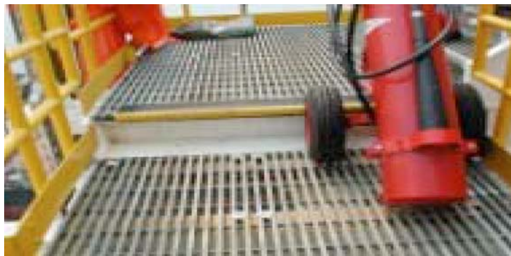
FIG. X1.8 FRP Grating Heavy Duty Nosing Bar
