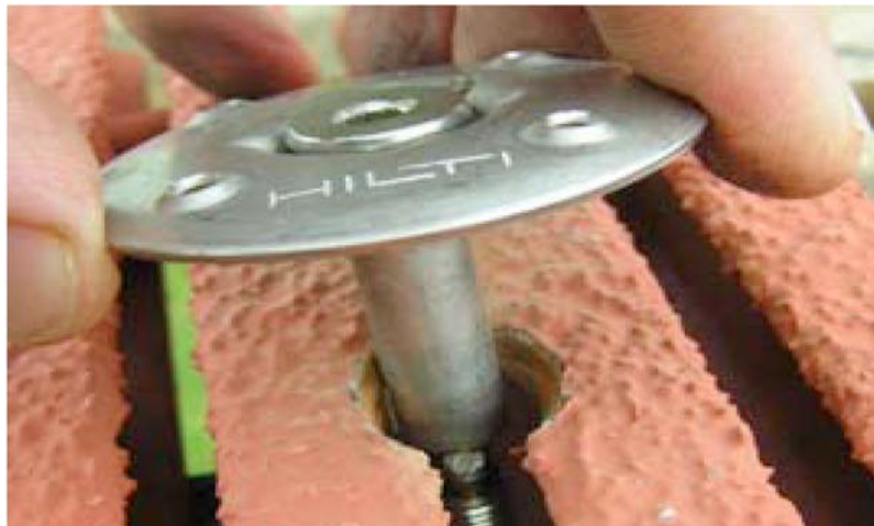
FIG. X1.12 Cut Edges of FRP Grating open to the Environment
