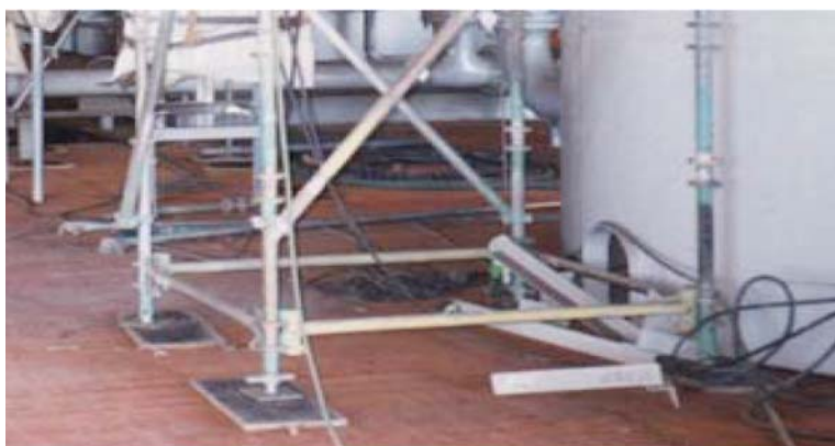
FIG. X1.15 Correct Distribution of Load on FRP Gratings
